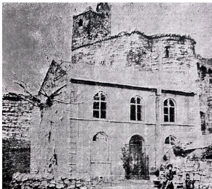
BETHESDA WELSH WESLEYAN CHAPEL (View taken shortly before its demolition in December, 1962)
